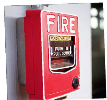
Fire Alarm Sensors Installation & Testing
